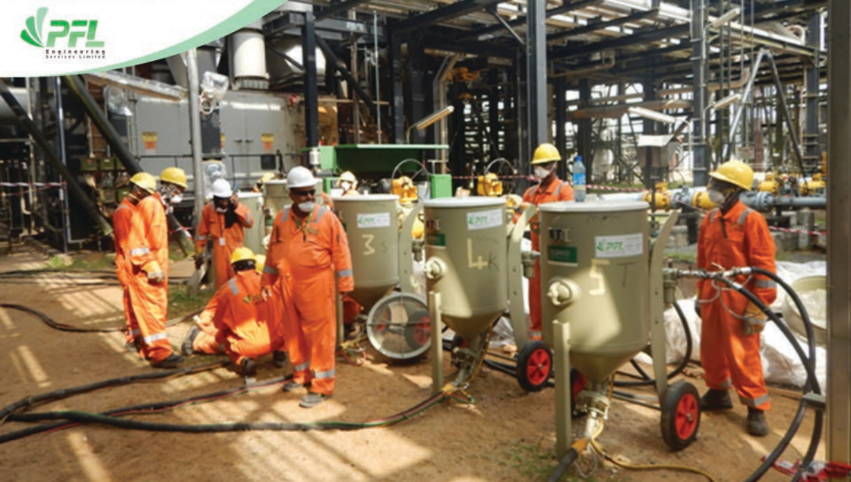
Blast Pots put to use at site
