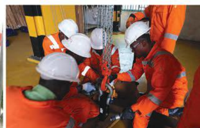
Lifting Operations Training
